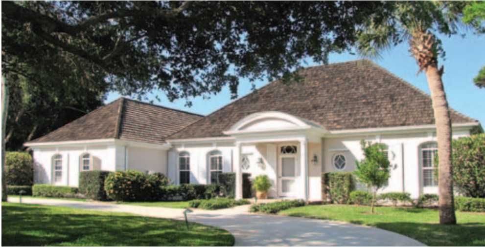
30 : 551 Indian Harbor Road : Enjoy stunning, private lake views from this charming 3BR+Den/5.5BA residence perfectly sited along the southeast corner of Indian Lake. Boasting 3,600± SF, features include a generous living room with beamed ceiling and fireplace, formal dining room with custom built-ins adjoining the expansive lanai, center island kitchen, den with full bath, and a private master suite with tray ceiling, built-ins and his and her baths. $1,675,000
